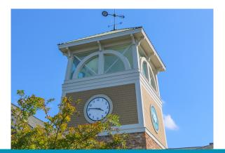
What we have now is a leaking tower that is weakened by the warping of materials, never built to specifications, not built with commercial materials, plus the risk of mold developing between the walls. Any strong storm with high winds could blow out the weakened windows, forcing an immediate remediation
